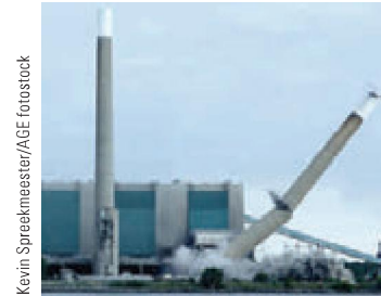
Figure 10.13 (Conceptual Example 10.5) A falling smokestack breaks at some point along its length.
